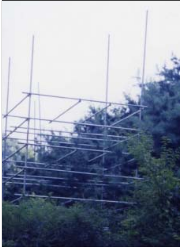
Fig. 11. Structural frame for the investigation of tree performance after crown shape control in age class II.
