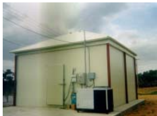
Fig. 64. The cold storage facility
