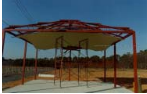
Fig. 60. Shape of ceiling of the dome-type cold storage facility
