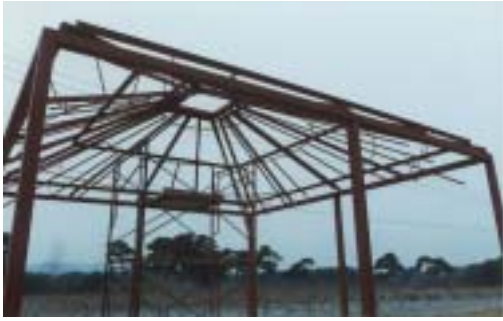
Fig. 59. Skeleton of the dome-type cold storage facility
