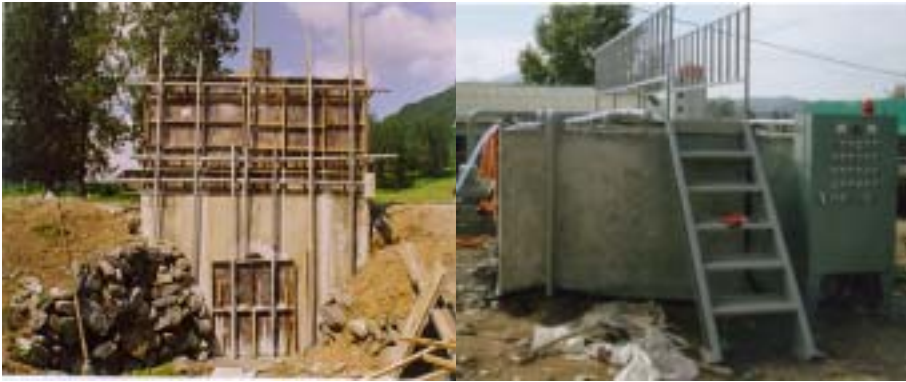
Figure 3-1-2. Photographs of construction site
