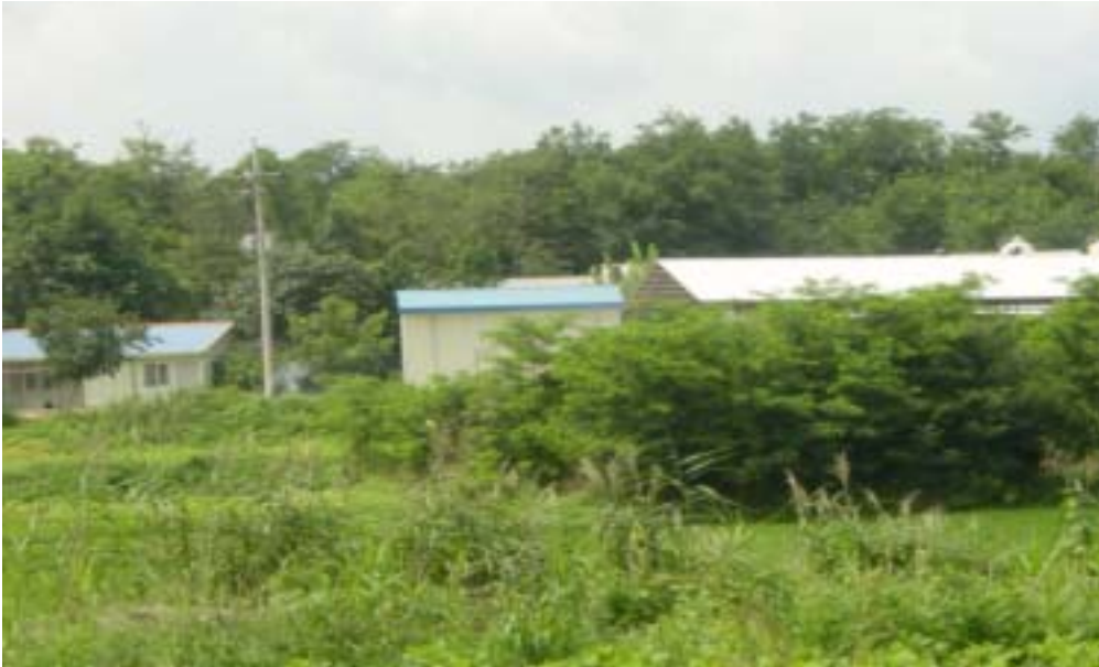
Figure 3-41. View of pig farm and two-stage ASBF system in containment
