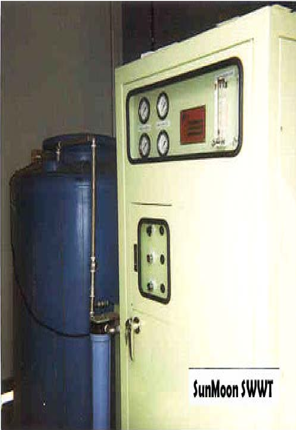
Figure 3-45. NF membrane system with control pane
