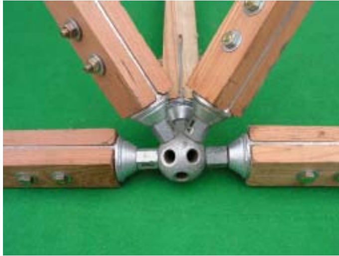
Fig. 7-6. Connector developed for wood space trusses
