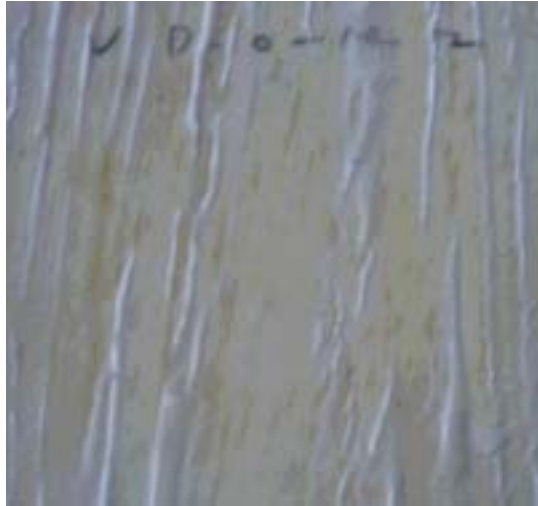
Fig. 5-120. Cracked appearance of laminated wood.
