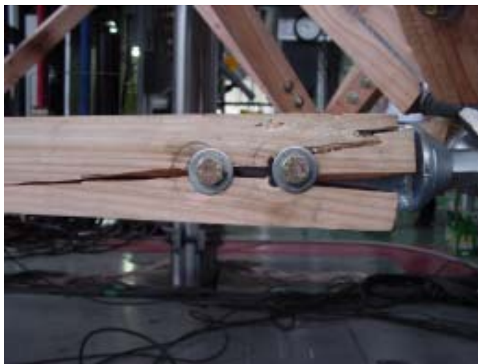
Fig. 7-20. Structural member failed at connector parts during full-scale test for wood space truss
