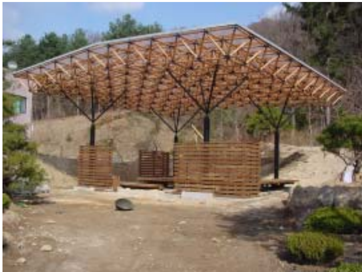
Fig. 7-45. Wood space truss structures fabricated
