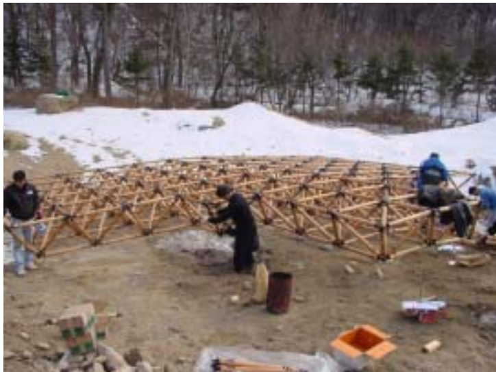
Fig. 7-41. Fabrication of wood space truss at construction site
