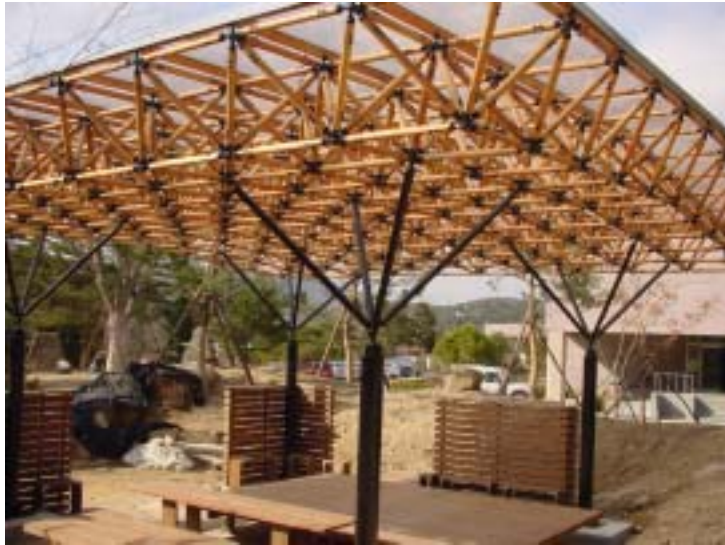
Fig. 7-44. Wood space truss structures fabricated
