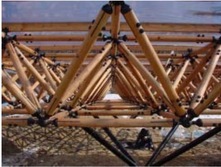
Fig. 7-42. Fabrication of connections for wood space truss at construction site
