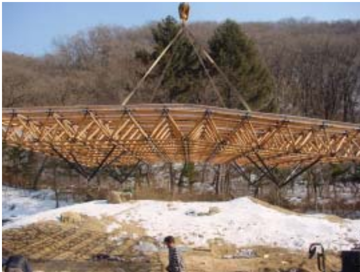
Fig. 7-43. Construction of wood space truss structures fabricated
