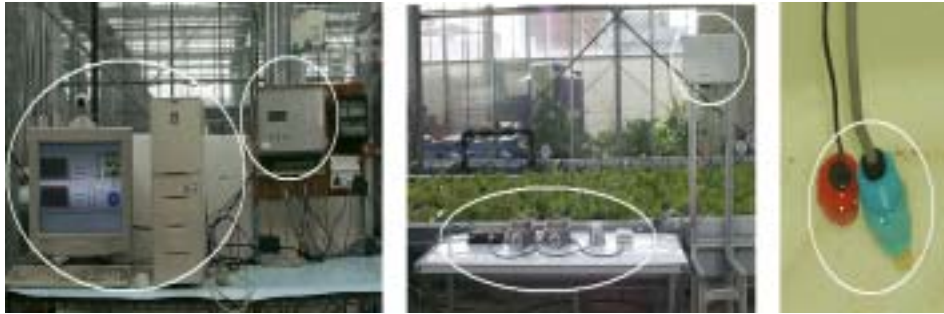
Fig. 5.10 Group Monitor, House Monitor and sensors in greenhouse I
