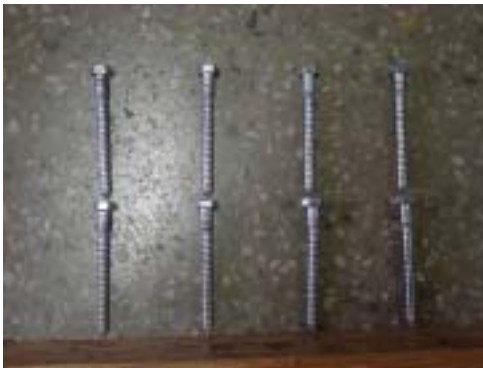
b) Deformation of lag-screw installed on top side
