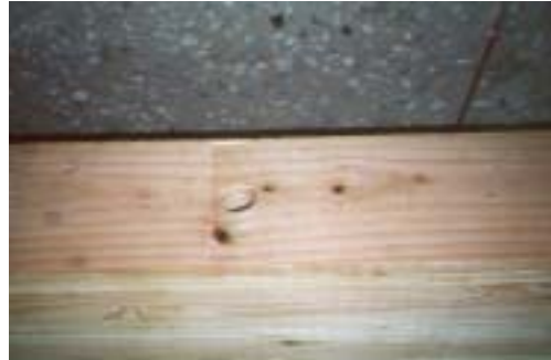
b) Deformation perpendicular to grain under scoop tie connector
