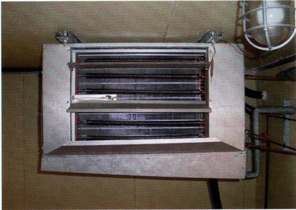
Fig. 42. Local installation of heatpump type- curing apparatus
