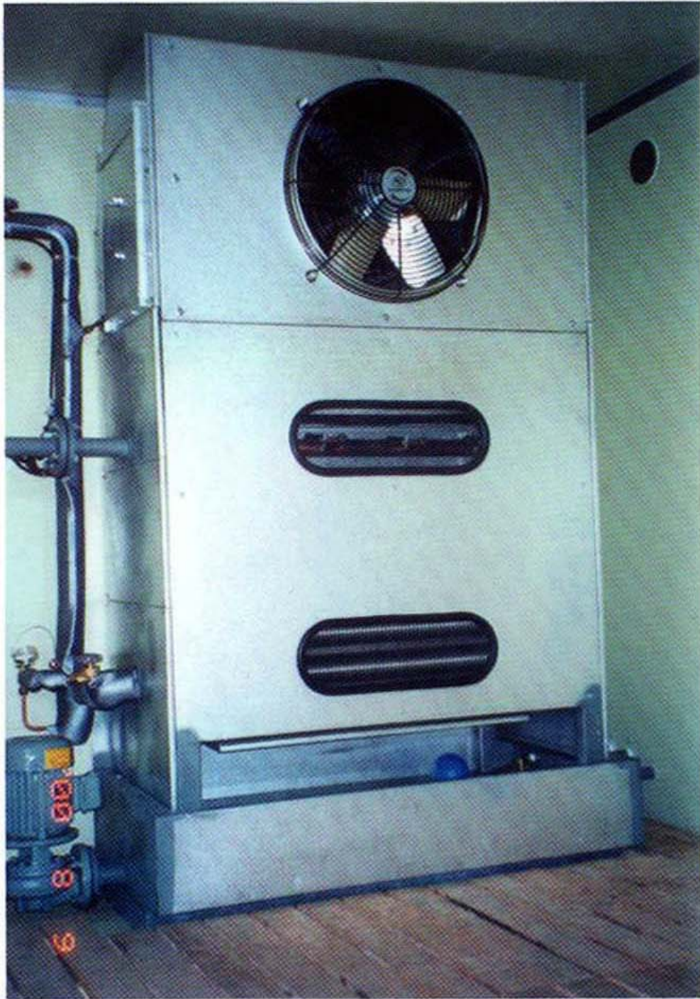
Fig.35. Installation of humidifying system in cold store.
