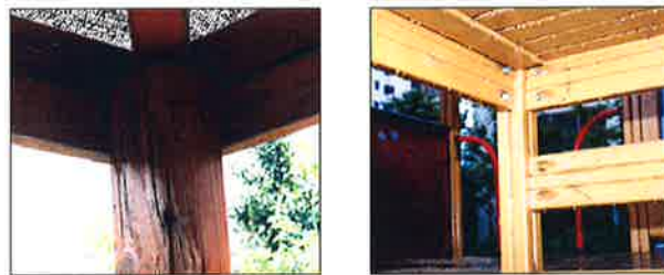
Fig. 2-6. The comparison of construction example for domestic and abroad company
