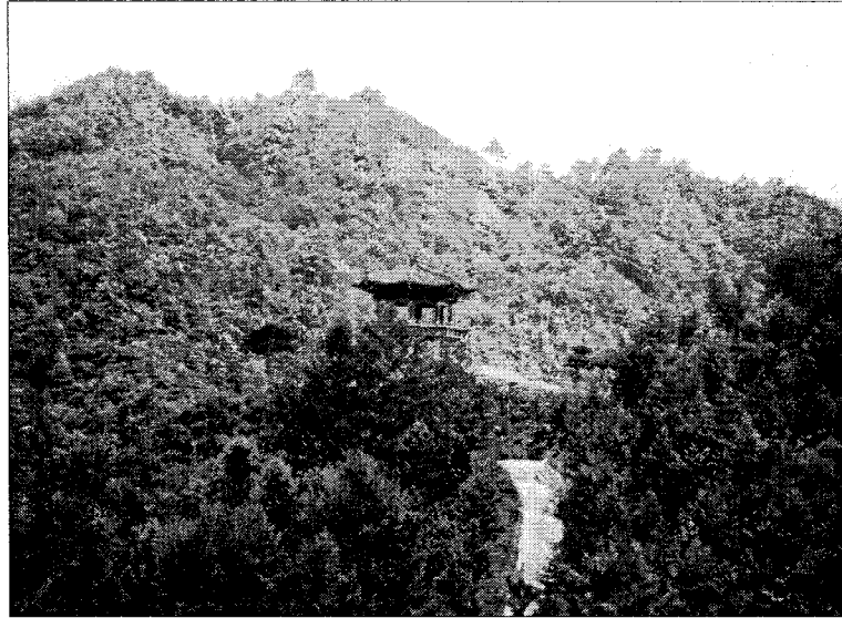
Fig. 2-69. The view of octagonal pavilion
