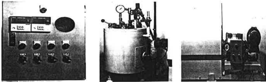
① Control panel ② Sulfur melting tank ③ Drum dryer part
