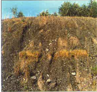
Photo 1. Eroded slope by destruction of restoration works.
