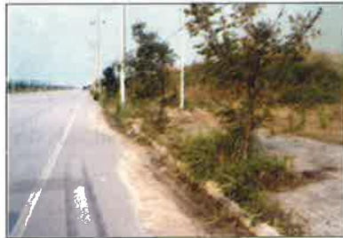
Photo 23. Street trees with salt damage.
