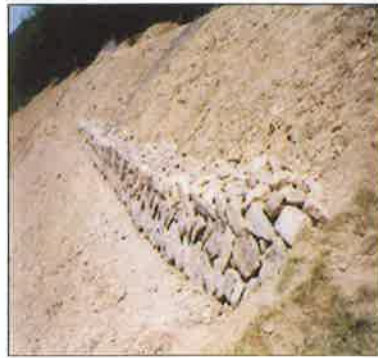
Photo 3. Stone masonry on slope(height 0.68m(left),height 0.51m(right)) (unimportant landscaping area)
