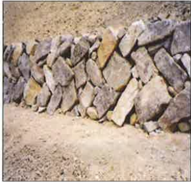
Photo 3. Stone masonry on slope(height 0.68m(left),height 0.51m(right)) (unimportant landscaping area)
