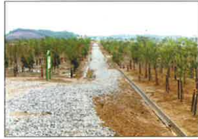
Photo 2. Soil-covering experiment site after construction.
