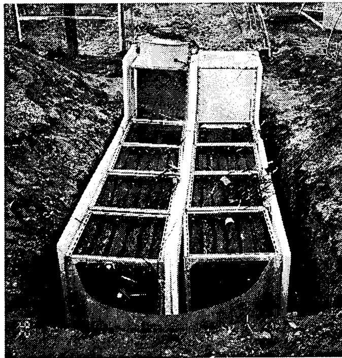
Fig 14(b) Photo of the underground latent heat storage system
