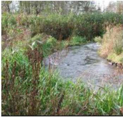
Location: Beckinghausen, Germany River: Lippe Type: pool-type bypass channel Slope: 1:30 to 1:35 Headloss: 3m Width: 3m to 6m Flow: 0.5 to 1m 3 /s Designer: Floecksmuehle Consulting Engineers Picture Source: Marq Redeker
