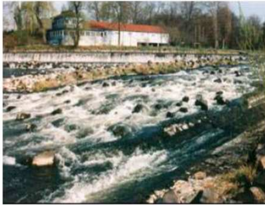
Location: Buisdorf, Germany River: Sieg Type: rock ramp fishway Slope: 1:20 Headloss: 2.65m Width: 15m Flow: 1.5m 3 /s Designer: StUA Köln Picture Source: Uli Dumont
