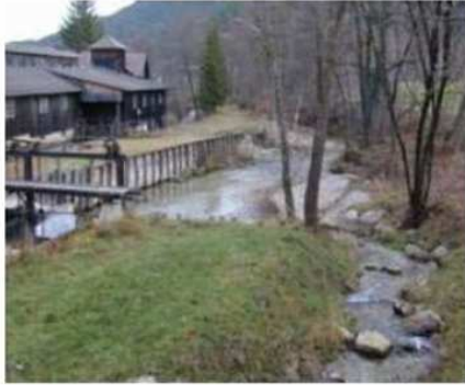
Location: Gutenstein, Austria River: Piesting Type: step-pool bypass channel Slope: 1:12 Headloss: 8in max at step, 5.5ft dam height Length: 65 ft Width: 5ft Flow: 1.5cfs (design), 30cfs (mean annual) Designer: EZB Picture Source: EZB
