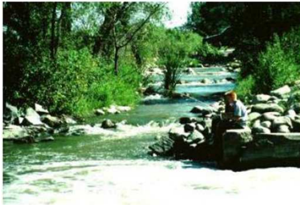
Project Name: Breckenridge Dam Fishway Location: Western Minnesota River: Otter Tail River Type: step-pool bypass channel Flow: 20 cfs during typical spring conditions Designer: Luthar Aadland, MN DNR Picture Source: Luthar Aadland
