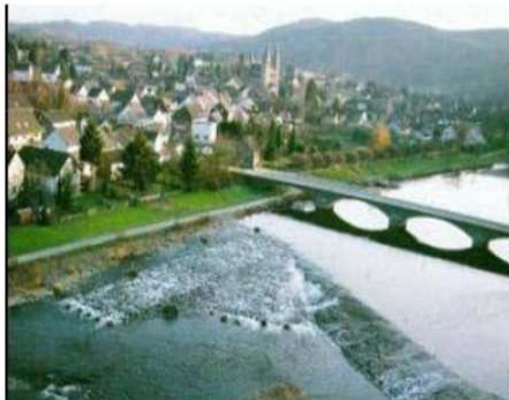
Location: Dattenfeld, Germany River: Sieg Type: rock ramp fishway Slope: 1:20 Headloss: 1.80m Width: 10m Flow: 2.0m 3 /s Designer: StUA Köln Picture Source: Uli Dumont
