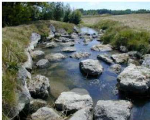
Location: Trautmansdorf, Austria River: Leithakanal Type: lowland bypass channel Slope: 1:143 Headloss: 4in max drop at step, 6ft dam height Width: 9ft Length: 765.5ft Flow: 0.7-18cfs (design), 100cfs (mean annual) Designer: Czeiner Picture Source: Piotr Parasiewicz
