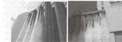
Fig 3: Actual photograph of ice layer formation of the general vaporizer
