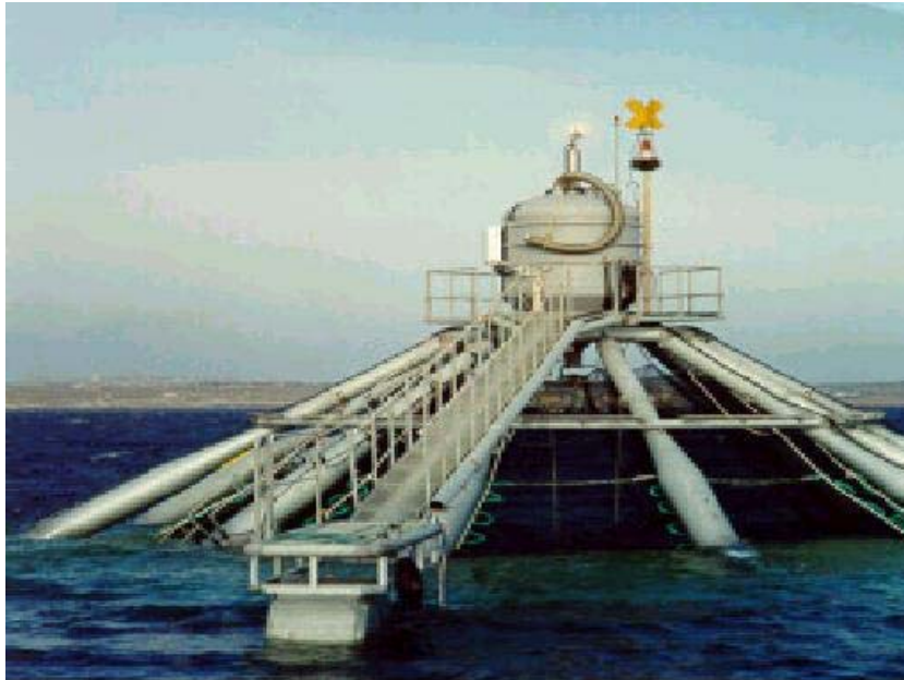
Fig. 4. fixed offshore aquaculture system.
