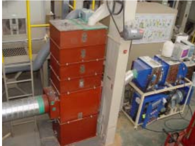
Fig. 3-20 View of drying test.
