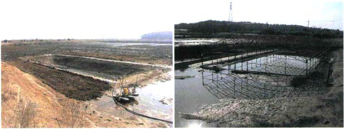
Fig. 71. Construction of wintering grounds in earthen pond.
