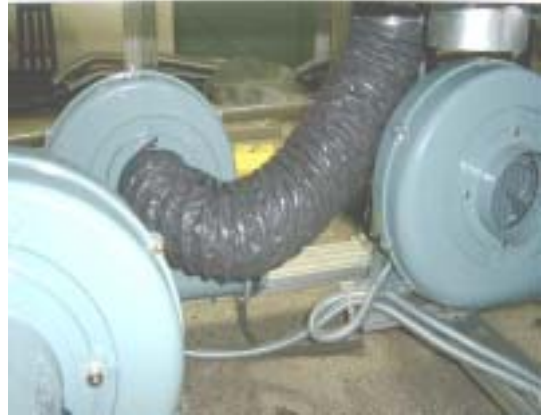
Photo. 57. After connecting blast fan & exhaust pipe.
