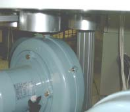
Photo. 56. Before connecting blast fan & exhaust pipe.
