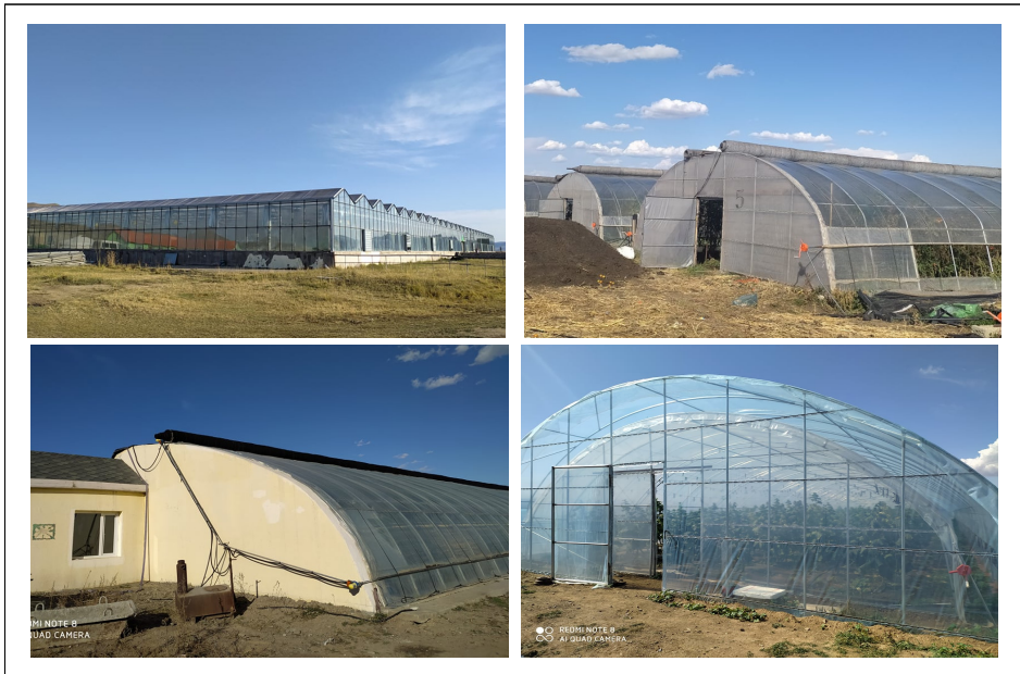
〈Figure 6〉 Greenhouse types in Mongolia. The first picture is a winter glass greenhouse (Tumen-suikh LLC); second picture is a blanket greenhouse; third picture is a Chinese-style solar greenhouse (Senjit-Oyu LLC); fourth picture is a double-layer greenhouse.
