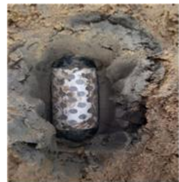
(c) Filling zone near conduit
