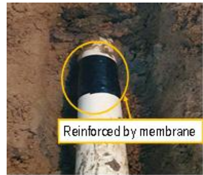
(c) Filling zone near conduit
