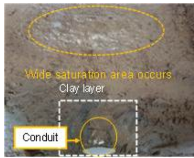
(b) Downstream slope
