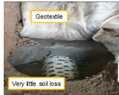
(c) Filling zone near conduit
