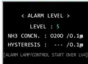
<Fig 4-15> ALARM LEVEL 5 설정
