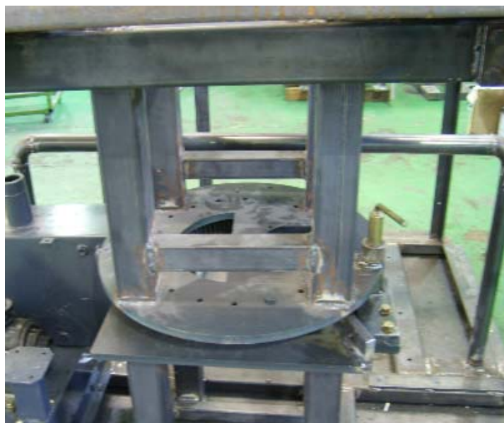
<Fig. 3-15> A rotation frame which has been mounted
