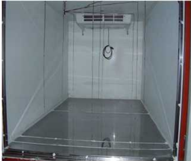
Photo 5 Temperature measurement at each point in refrigeration box.
