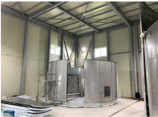
(c)버퍼조 100ton 설치(외부)-1
