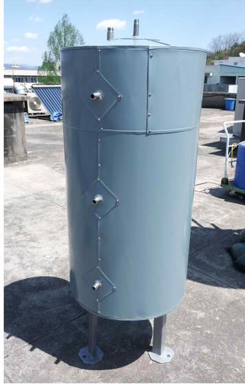
Figure 1-19. Small size of thermal storage tank.
