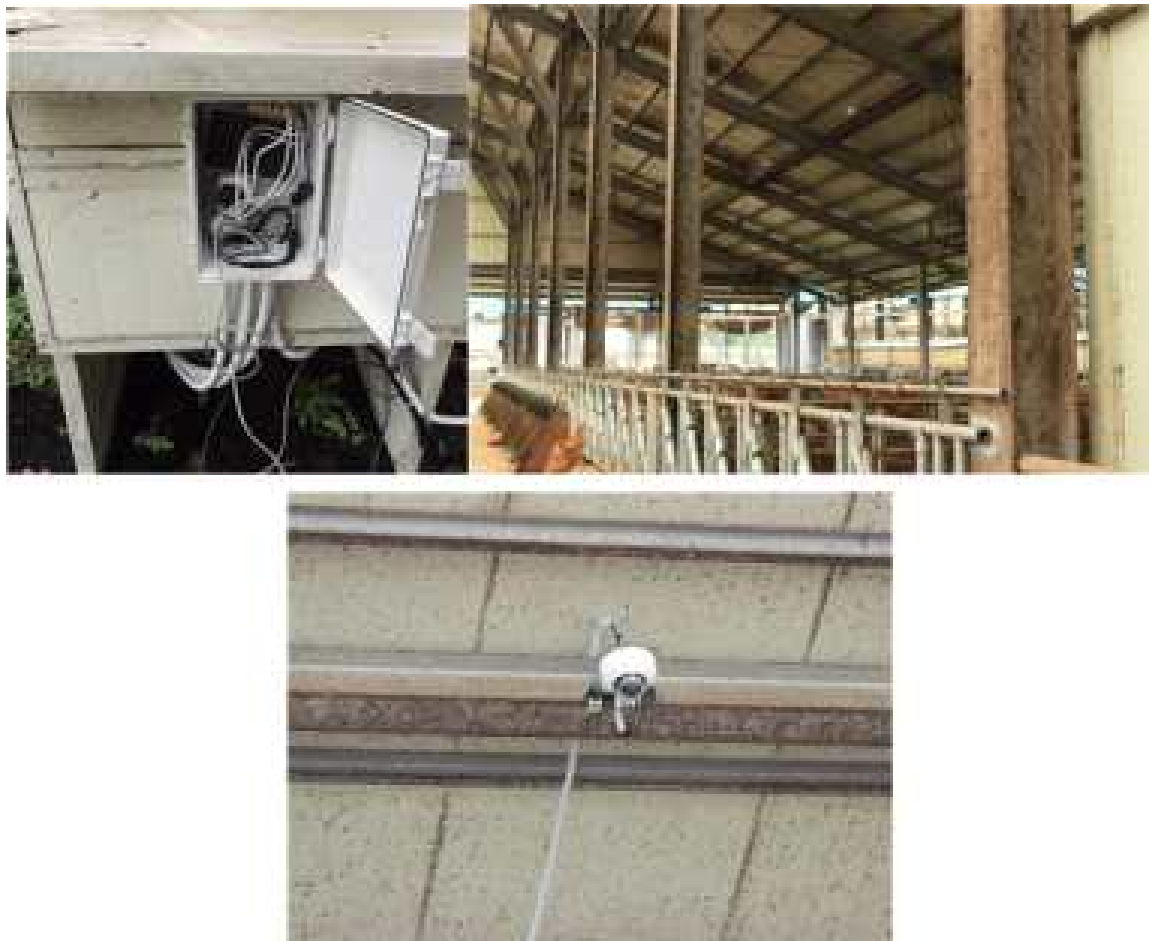
그림 1-56. Installed gateway, camera, environment measuring device in inside the farm
