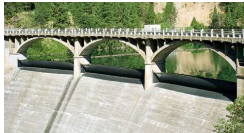
(h) Crest Rasing (USA, Pit 3 Dam)
