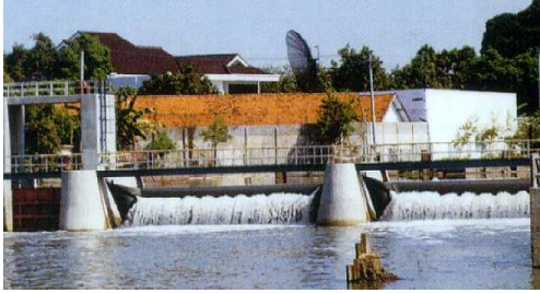
(c) Water Supply (Indonesia, Gubeng Dam)
