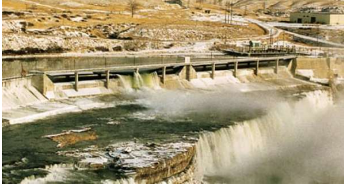
(a) Hydro Power (USA, Rainbow Dam)
