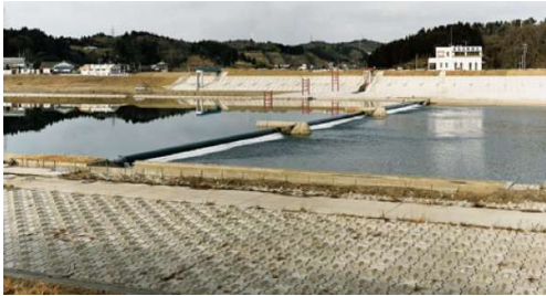
(e) Tidal Barrier (Japan, Naruse River)
