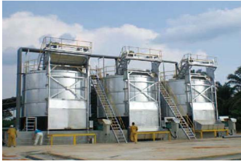
<그림-12> Fermentation equipment for composting animal waste and raw garbage
