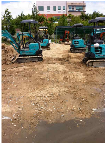
Figure 118 Unpaved test ground
