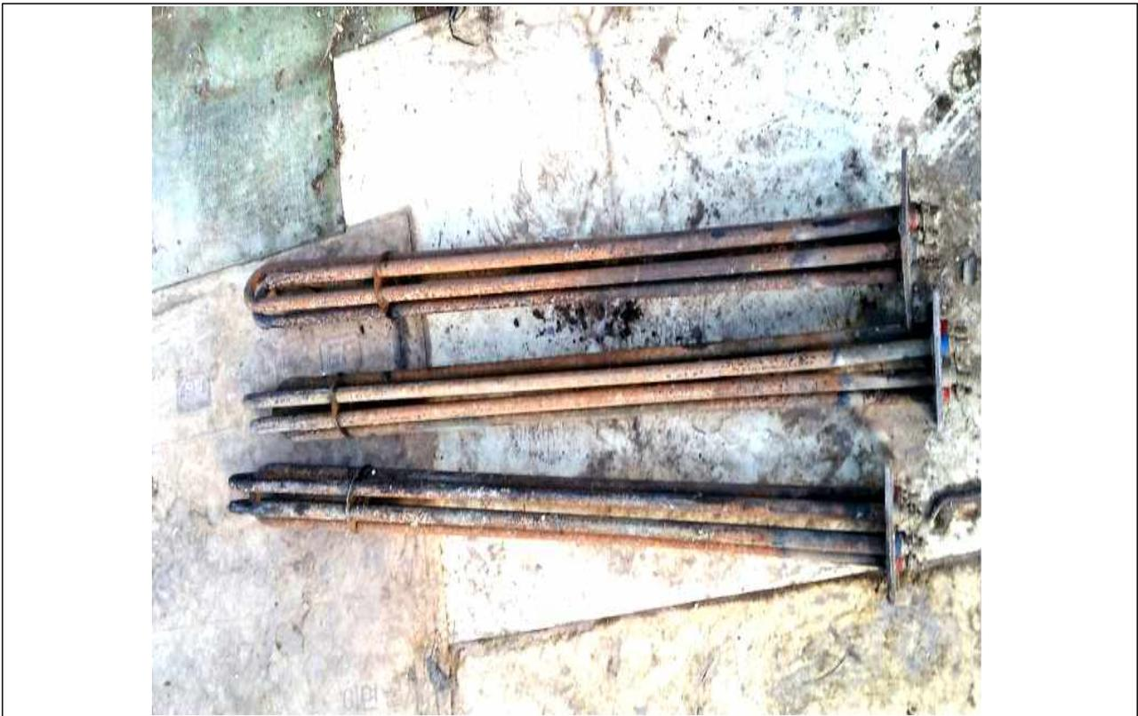
Figure 17. High-capacity sheath heater photo for current K boiler heating
