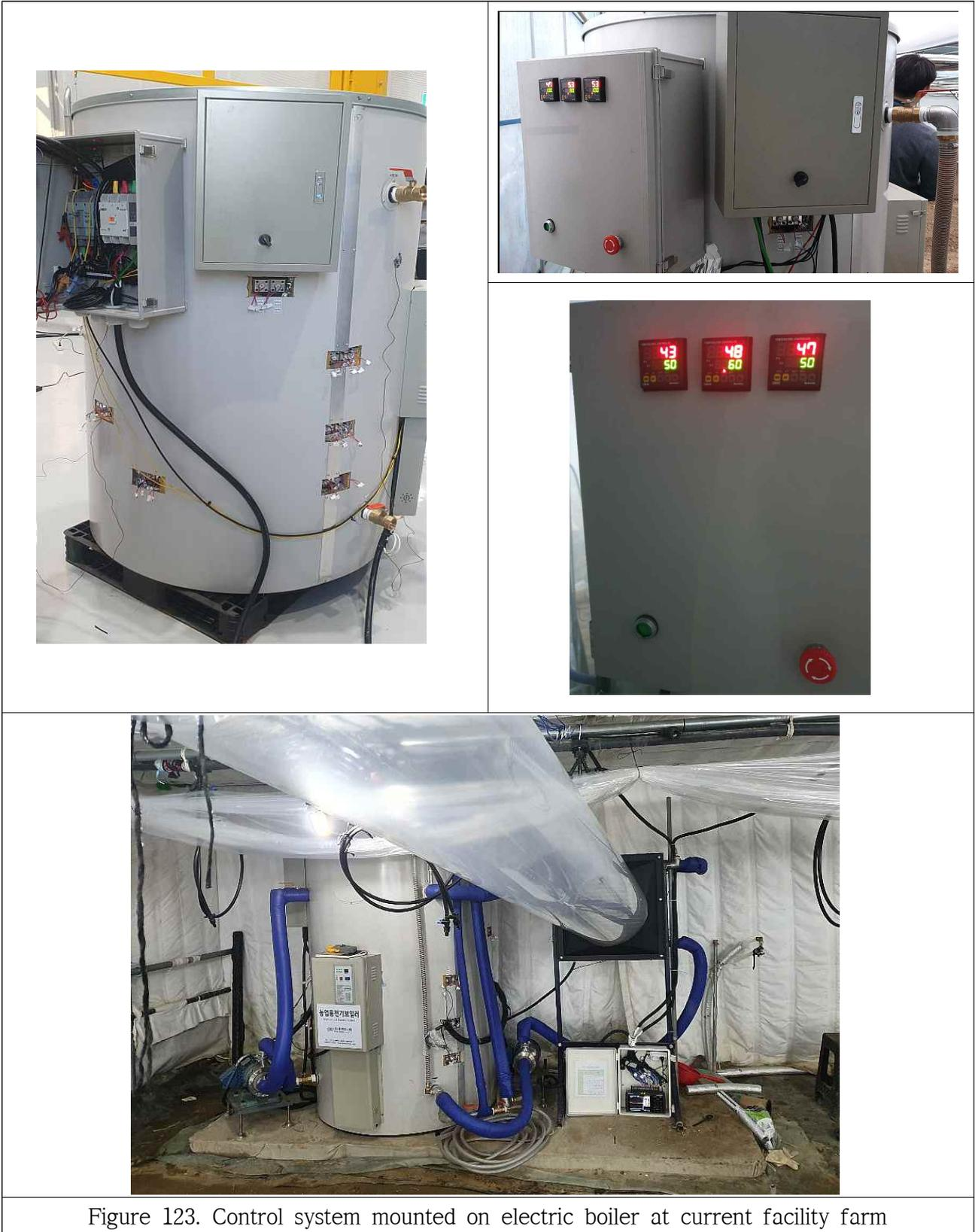
Figure 123. Control system mounted on electric boiler at current facility farm
