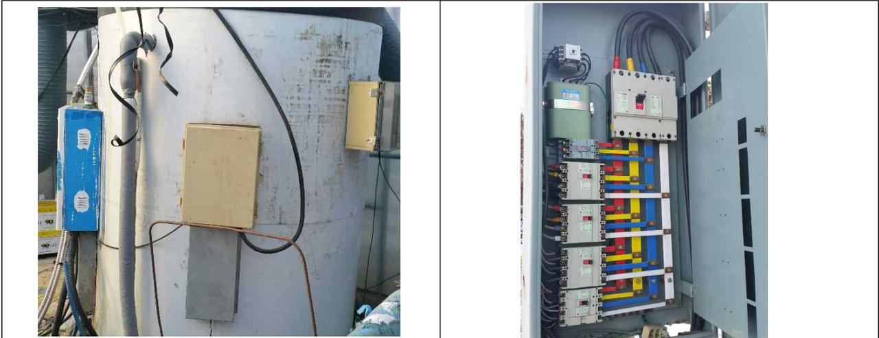
Figure 78. Control system mounted on electric boiler at current facility farm
