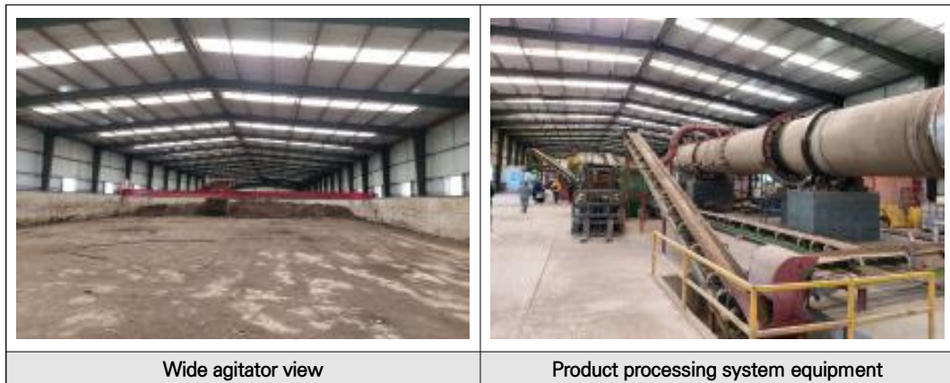
<Figure 2-2> Indoor fertilizer production plant (Mongolian Eco-Fertilizer LLC)
