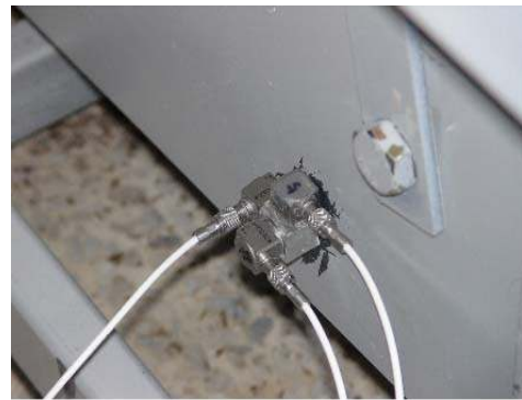
Fig. 3-6. A picture of acceleration sensors attached to the preliminary sterilizer.
