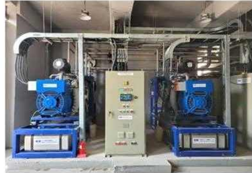
열병합발전기 : CHP (Combined Heat and Power)
