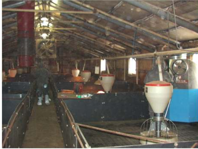
Fig. 16 Pig house A with one wet air cleaner
