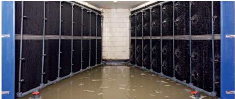
Front view of the filter; a nozzle group sprays water onto the filter at intervals
