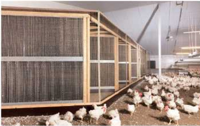
Use of the StuffNix dust filter in a broiler breeder house
