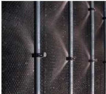
High-quality plastic pads are sprayed with water → dust does not adhere
