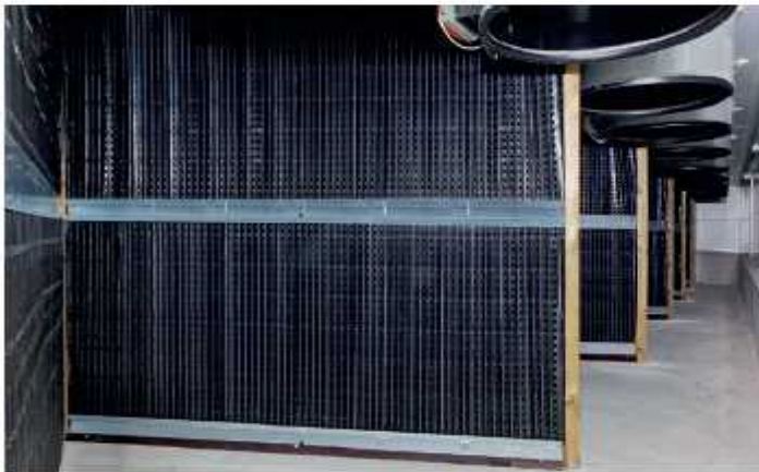
Back view of the filter; fans suck the exhaust air through the filter
