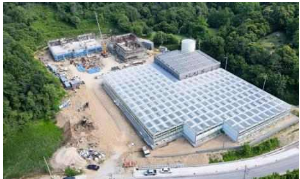
Under construction of test-site greenhouse (4)
