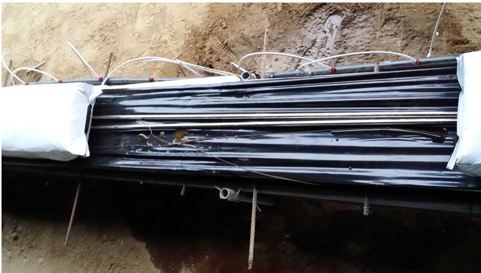
Fig. 55 Installation of BJTHP(stainless steel)
