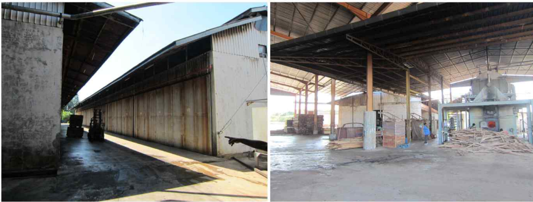
Figure 3-9. Kiln drying system for laminae in MY-B
