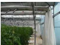
그림. 2. Thermal screens and hot air heating system in experimental greenhouse
