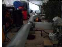
그림. 2. Thermal screens and hot air heating system in experimental greenhouse
