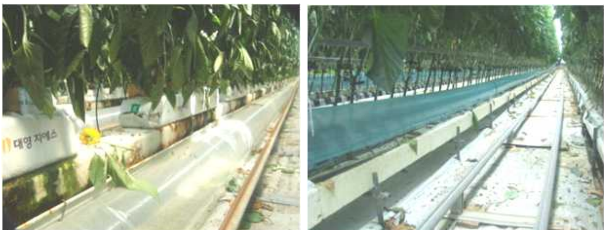
[그림 3-I-15] Using methods of air duct facility in paprika's green house.
