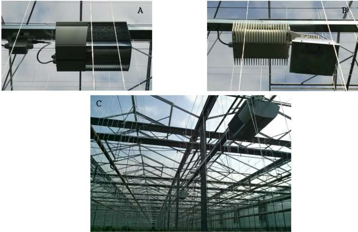
[그림 3- I -20] Photos of high pressure sodium (HPS, A) and lighting emitting plasma (LEP, B) lamps supplied for this research, and two lamps set in green house (C).
