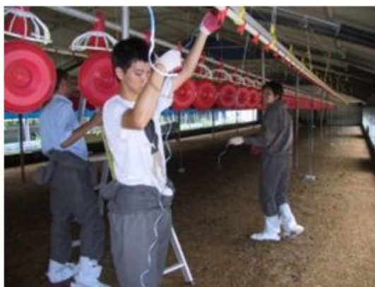
Fig. 3.1.3. Installing of Hobo sensors
