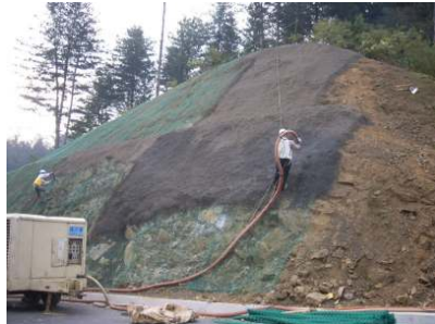
(e) Installation of Nok
