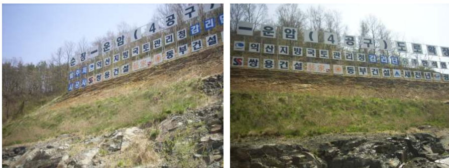
Figure 50. The landscape of the 1st field feasibility test site, April 2008.
