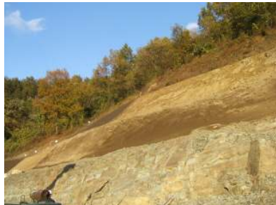
(f) Installation of BA-native
