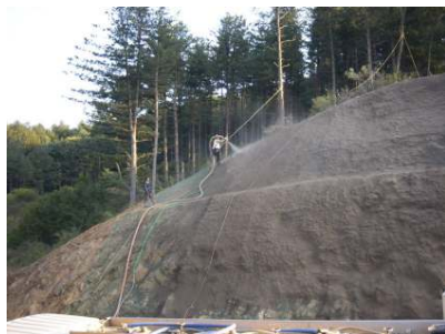
(g) Installation of BA50
