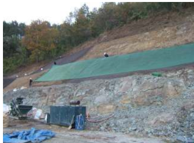
(h) Installation of plastic mulch
