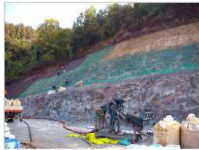
(b) Installaton of wire net
