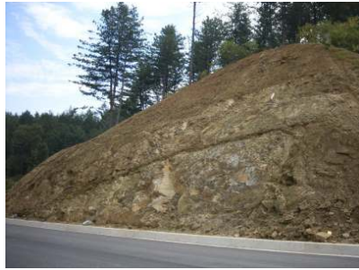
(a) Before intallation
