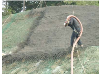
(f) Installation of BA10
