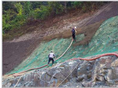
(c) Installation of Nok-grass
