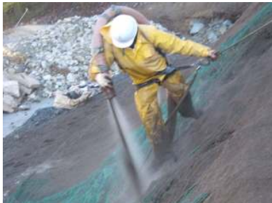
(e) Installation of BA-native
