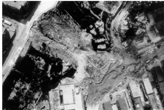
(a) The Sau Mau Ping landslide
