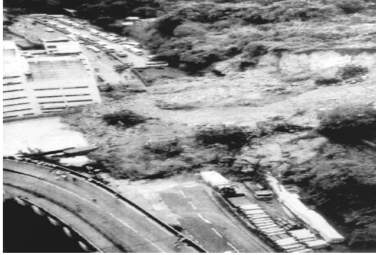
(e) The Fei Tsui Road landslide
