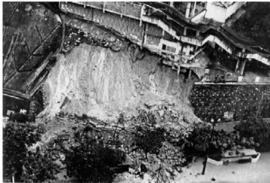
(c) The Kwun Lung Lau landslide
