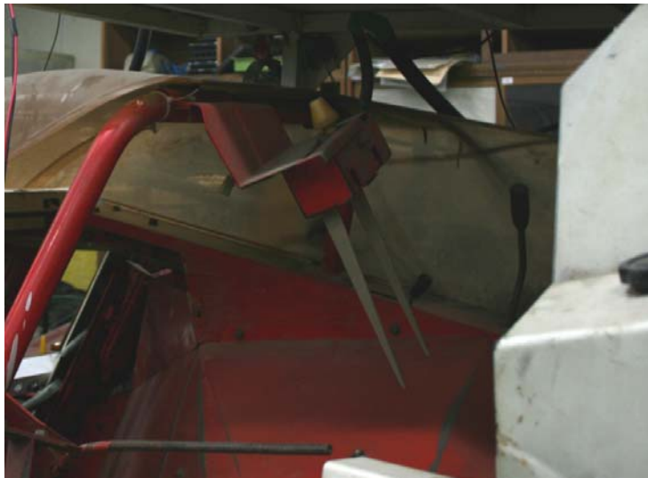
Fig. 1.8 Installation of limit switch
