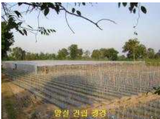
Net house construction
