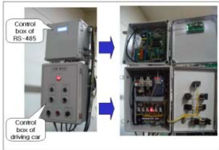
Fig. 21 Surface and inside view of RS485 and driving car control box.
