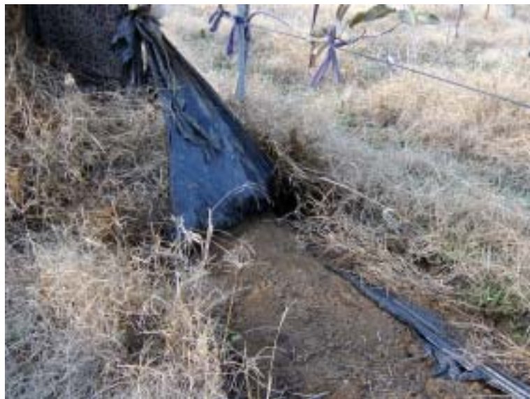
Fig. 3 A work of vinyl removal
