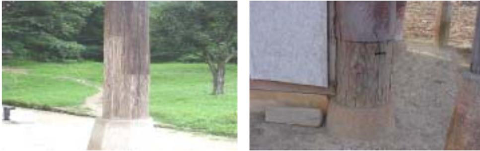
**Fig.16. Deteriorated supporting post in 'dongbari' connection.**
