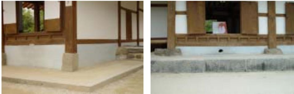
Fig.15. Examples of fully closed crawl space and closed crawl space with ventilating openings.
