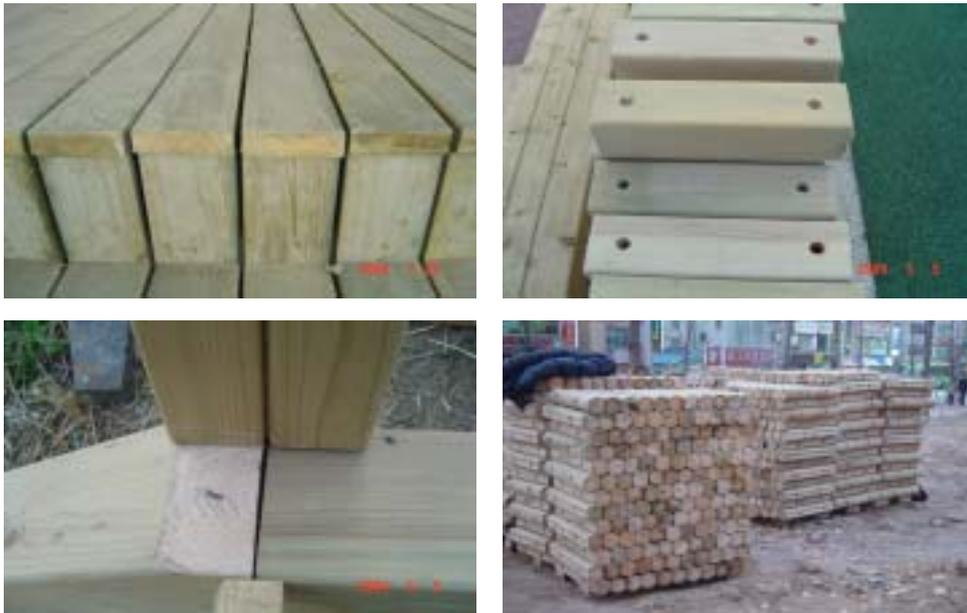
**Fig.21. Untreated interior exposed by cutting or boring of preservative-treated wood at construction site.**
