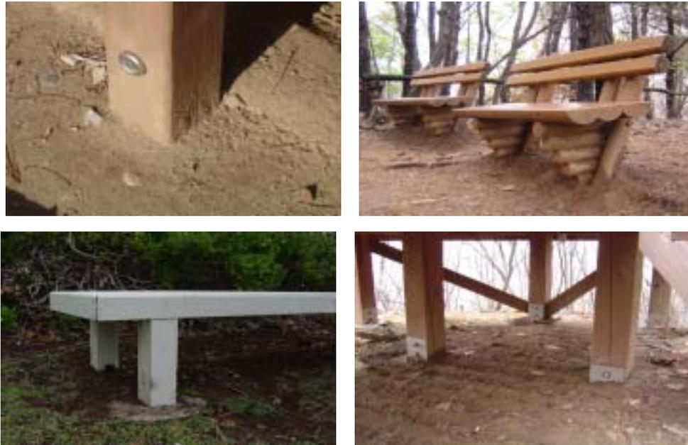
Fig.19. Ground contact uses of untreated and surface-coated wood.
