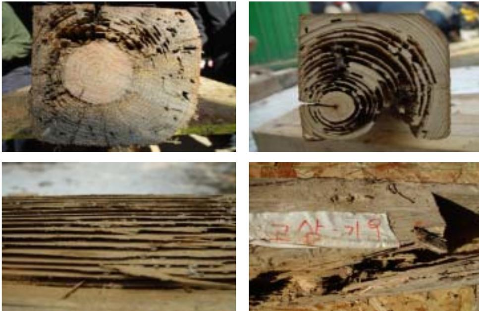
**Fig.6. Typical termites damages observed in dismantled wood members of old wooden building.**
