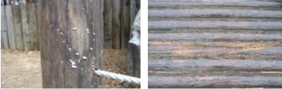
**Fig.20. Decay damages of preservative treated wood due to poor preservative treatbility.**
