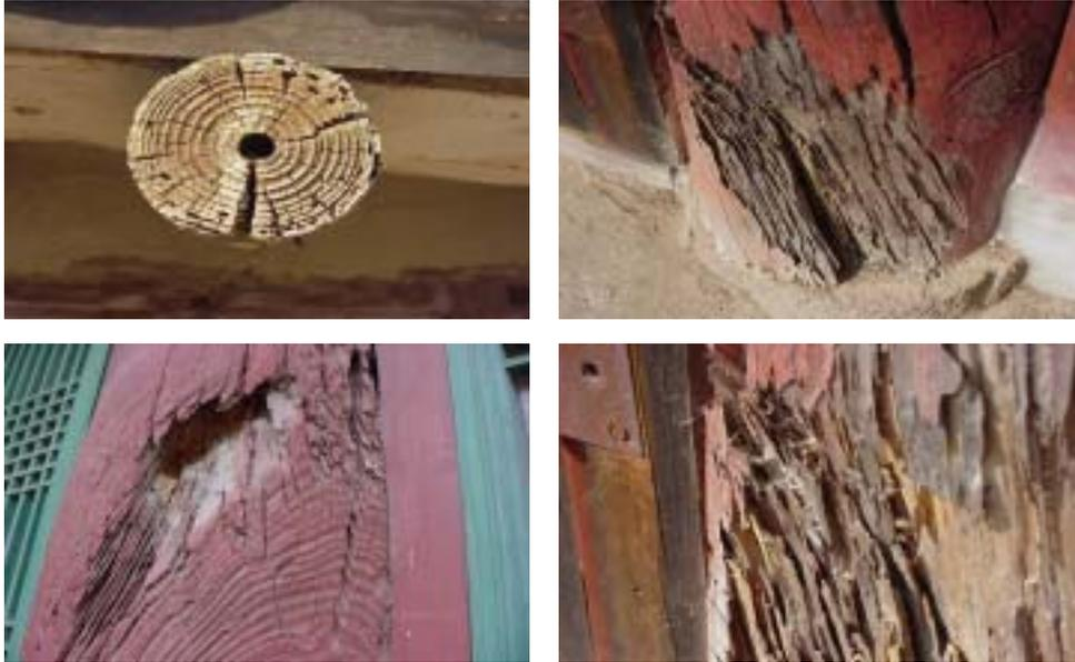
Fig.9. Typical termite attacks observed in old wooden buildings.
