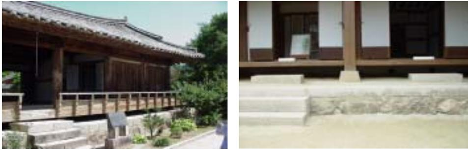
Fig.14. Examples of open crawl space under floor.
