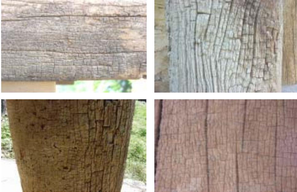
Fig.7. Typical soft rot damages observed in old wooden buildings.
