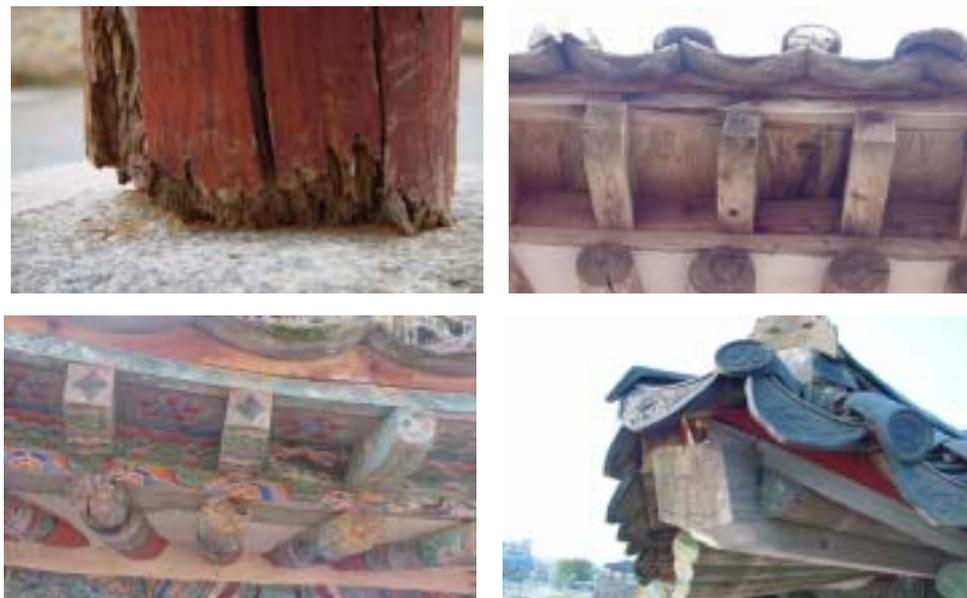
Fig.10. Decay damages of wood members by increased moisture contents due to direct rain wetting.
