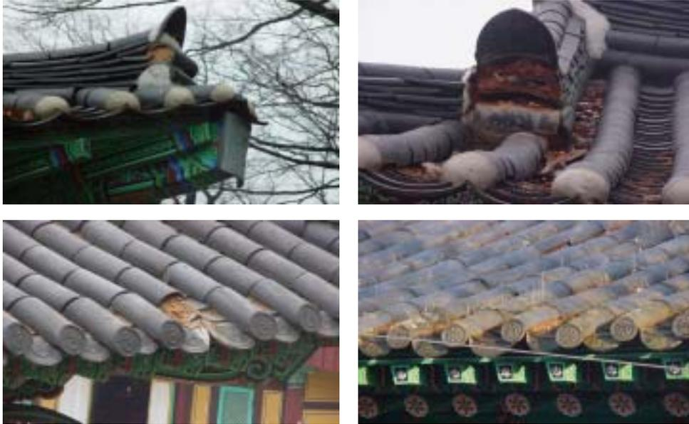
**Fig.12. Various examples of roof tile's breakage.**
