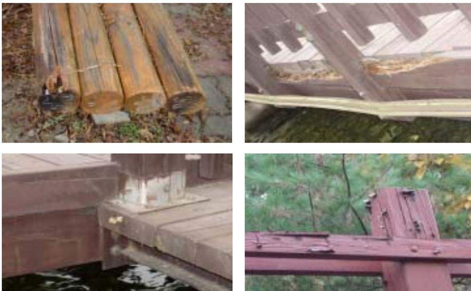
Fig.18. Decay damages of surface-coated wood with various film-forming and penetrating finishes.
