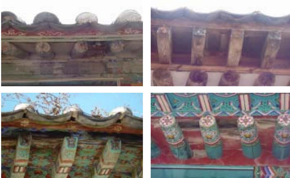
Fig.11. Decayed and discolored rafters due to rain seepage through roof.
