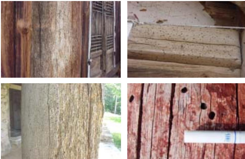
Fig.8. Typical insect damages observed in old wooden buildings.
