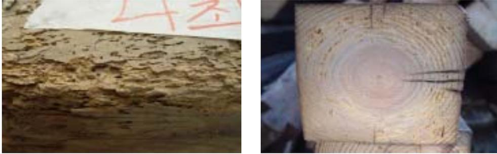
**Fig.5. Typical insect damages observed in dismantled wood members of old wooden building.**
