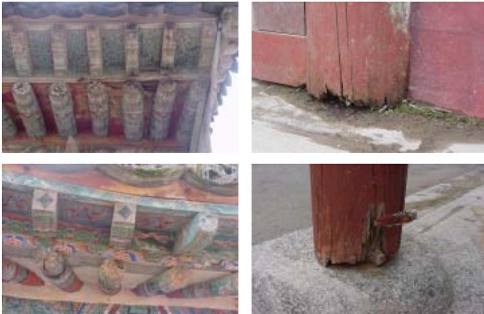
Fig.6. Typical decay damages observed in old wooden buildings.
