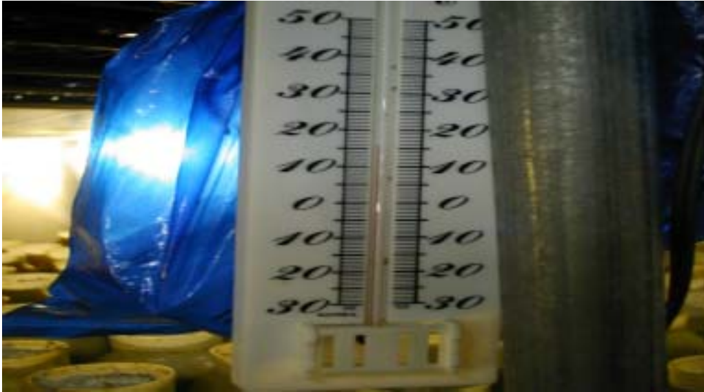
Photo 2-4. View of a thermometer for inside temperature instrumentation.
