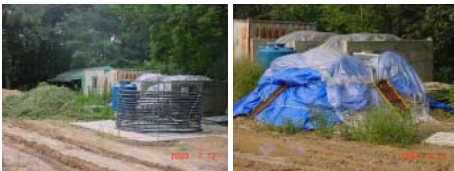
Fig. 4. Pipe installation(left) for hot water and fermenting bed (right)
