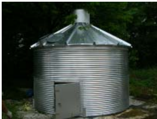
Fig. 30. Prototype Silo of Industrial Heat Exchanger
